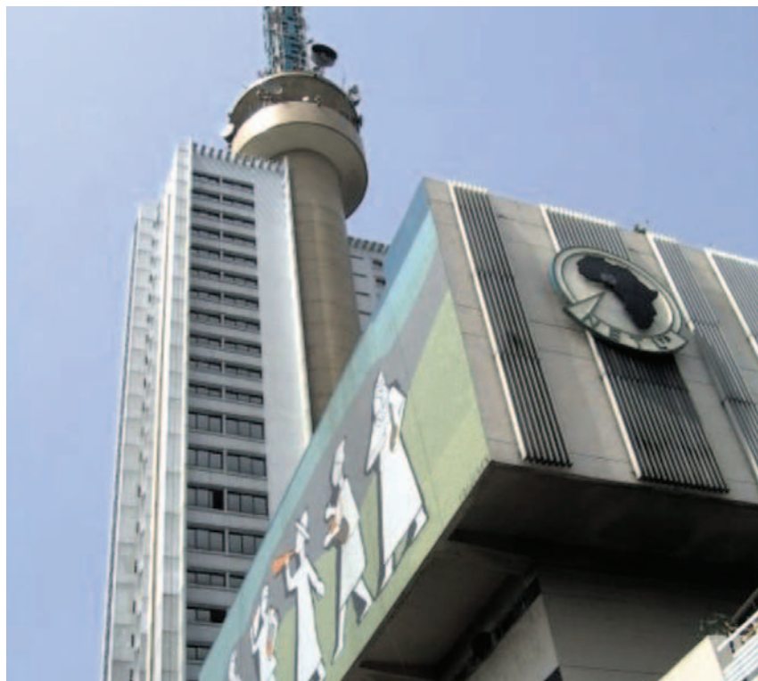
Part view of old NET building under refurbishment
